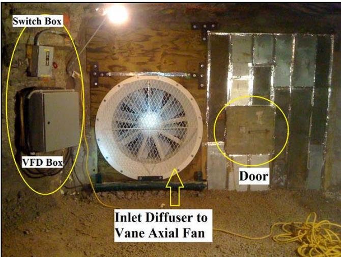
Figure 3. Electrical components at the West booster fan.
